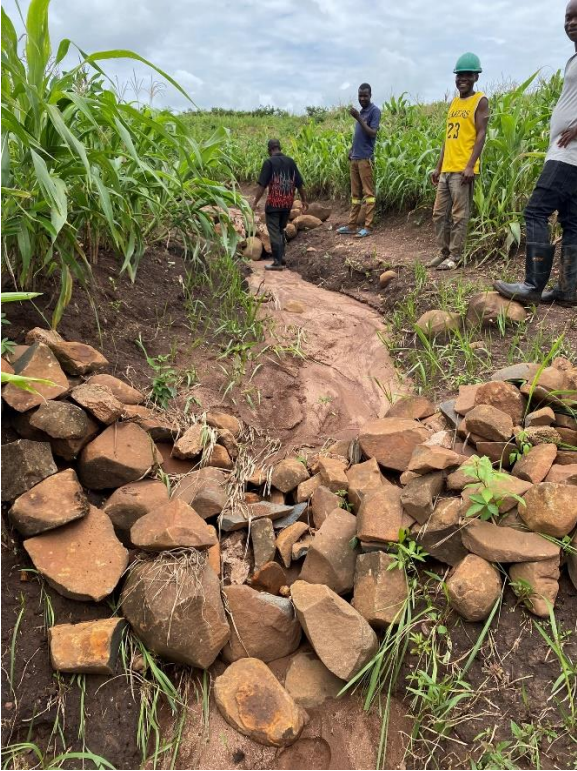
Constructed Marker Ridges and check dams at Sikoya to prevent erosion
