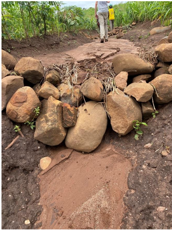
Constructed Marker Ridges and check dams at Sikoya to prevent erosion
