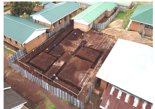
Δ Eye theatre under construction
