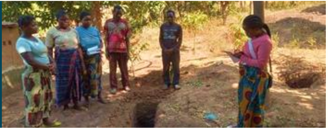
Supervisors at a site of latrine construction
