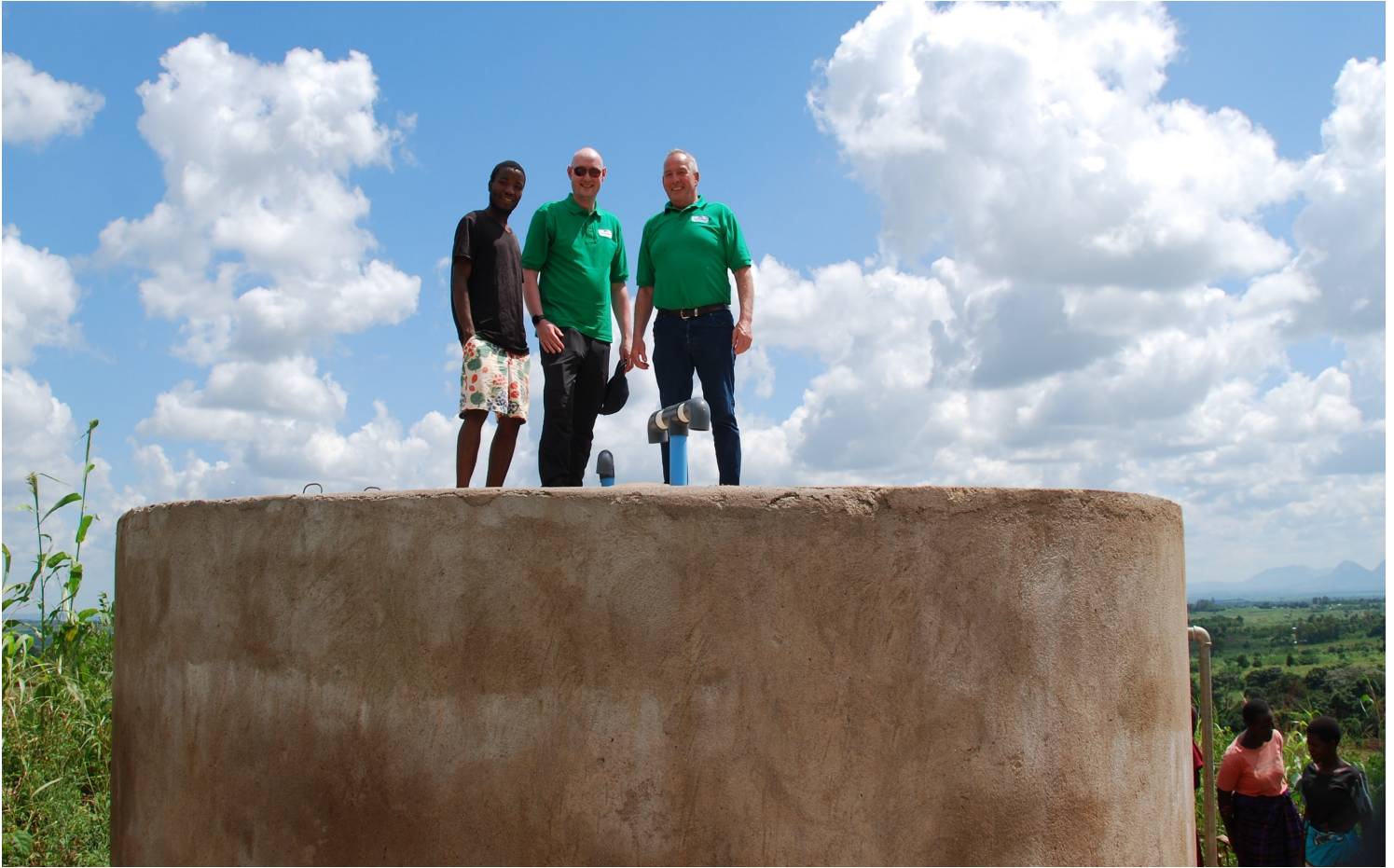
John Best and Ronan McCanny from Fane Valley inspecting the new Sikoya Irrigation Scheme
