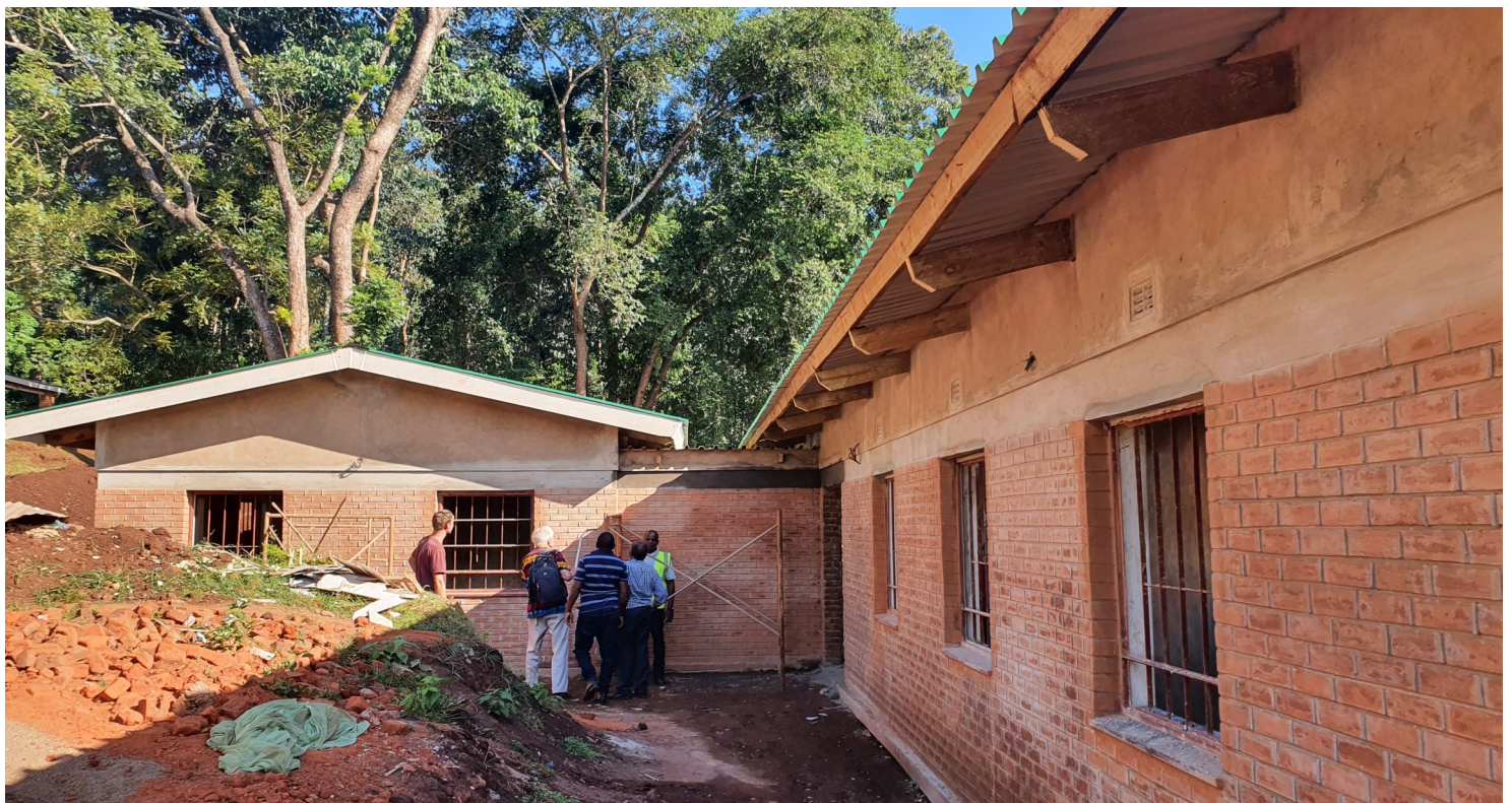
▲ Eye and physiotherapy building in progress
