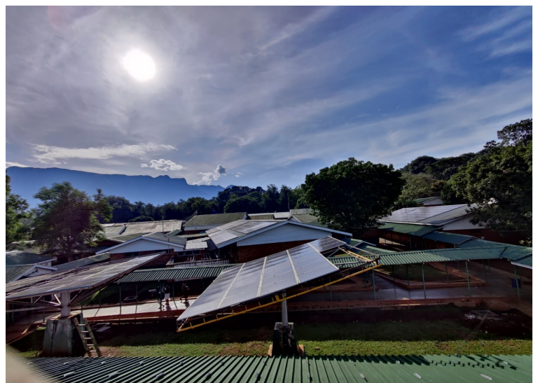
▲ Renovation of the solar trees
