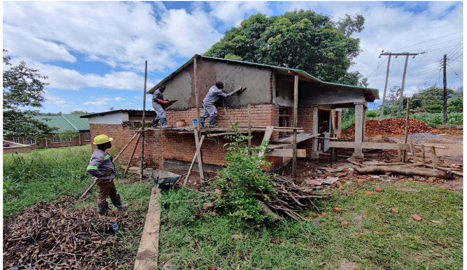
▲ Works in progress
