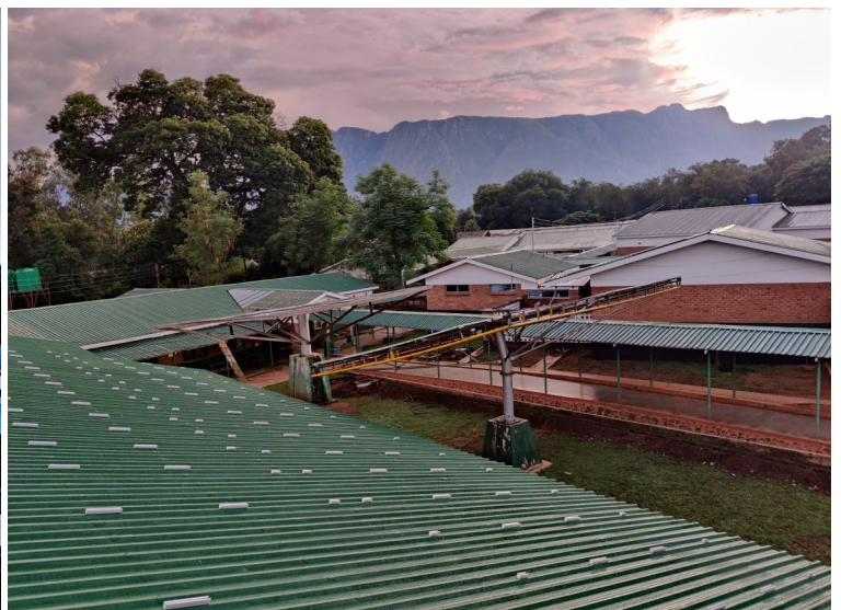
▲ Preparation for new panels on female ward
