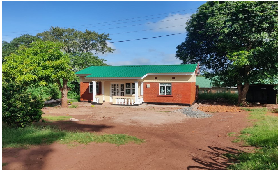
▲ The renovated house!
