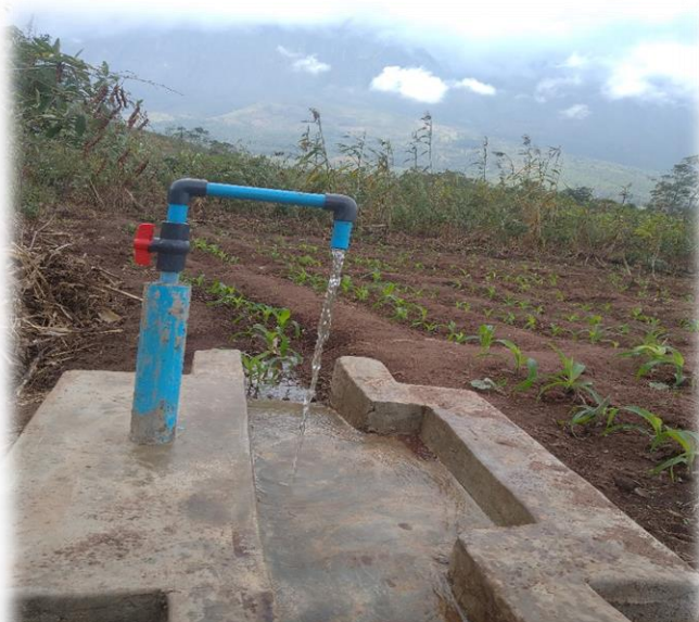
Picture 2: Mwanamvula irrigation scheme
