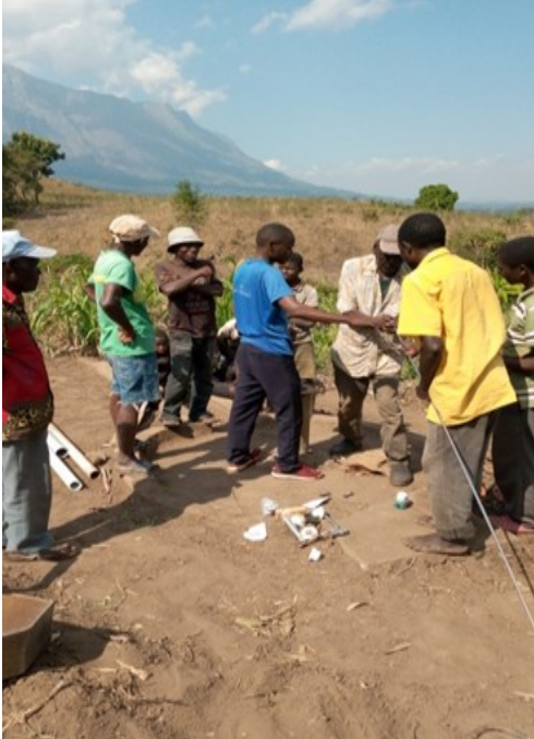
Namijingo borehole maintenance
