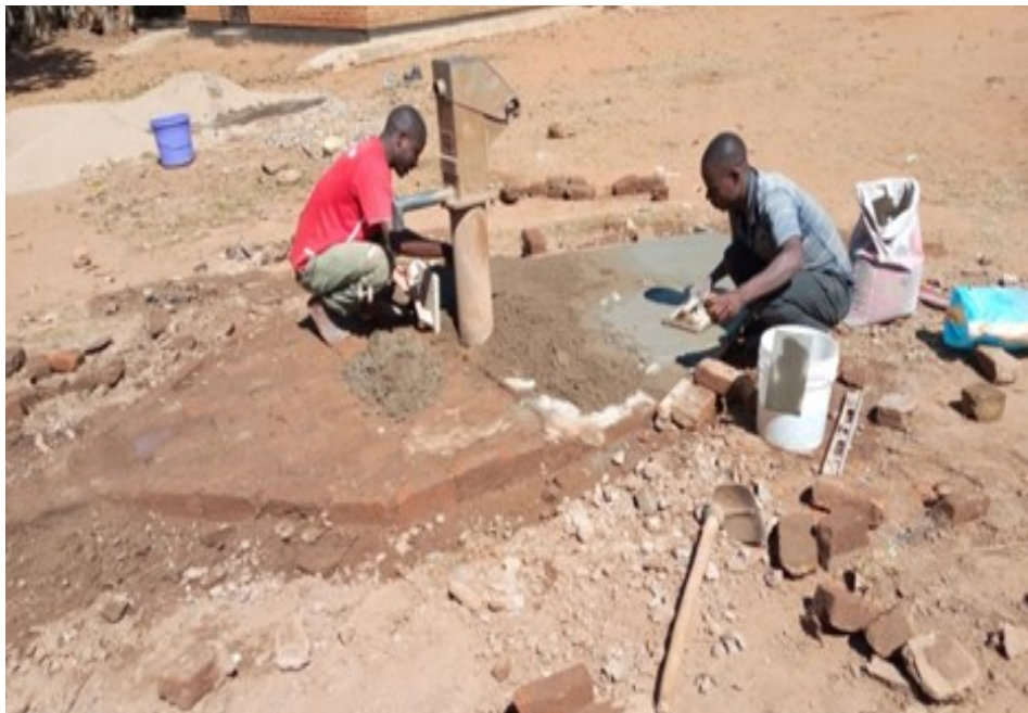
Borehole maintenance at Salamba village
