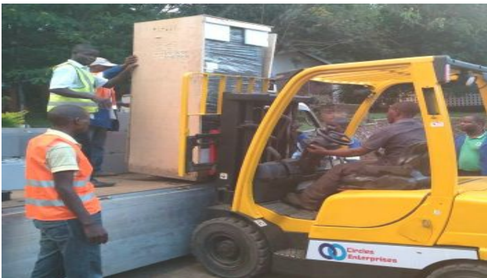
Moving new solar equipment into place has been quite challenging ▲
